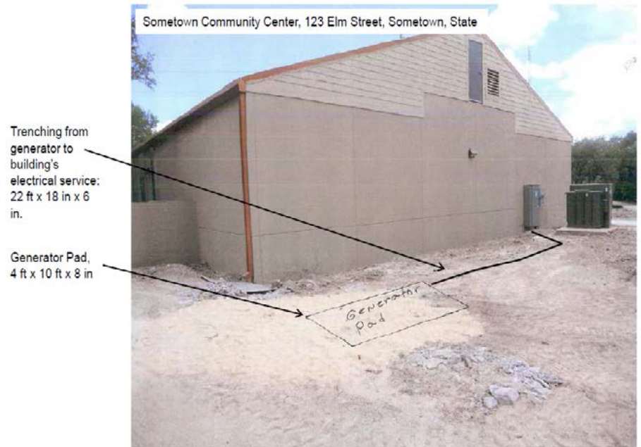
Figure 4. Ground-level photograph showing proposed ground disturbance area.
